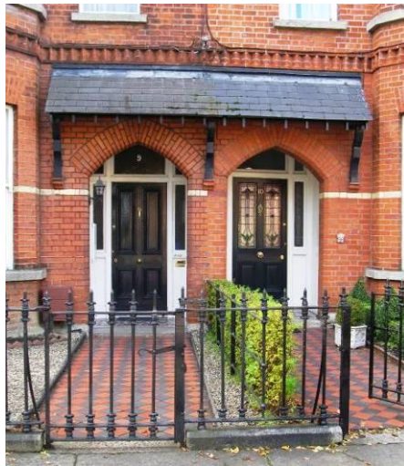
Paired porch entrance doors
